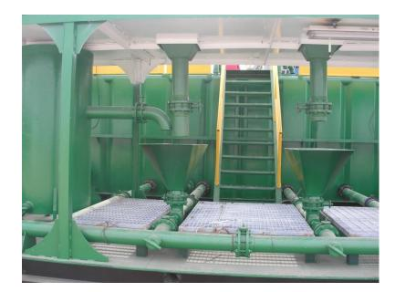
ALL TRANSITION AND LINKING PIPES SCHEDULE ARE A 106-SCH 80 ALL BUTTERFLY VALVES ARE FROM SANAM'S PRODUCTS DRESSER SLEEVES PRESSURE RATINGS ARE 1000 PSI HAMMER UNIONS PRESSURE RATINGS ARE 2000 PSI TANK SIDES AND SKIDS PLATES ARE ST-52 FLANGES AND PLUG VALVES ARE FROM CLASS 150 GALVANIZED CHECKERD GRATINGS WITH 4CM STRAPS AND 6X5 THICKNESS
